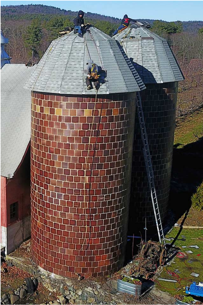
Left: Quonquont dairy barn silos roof replacement, 2020
