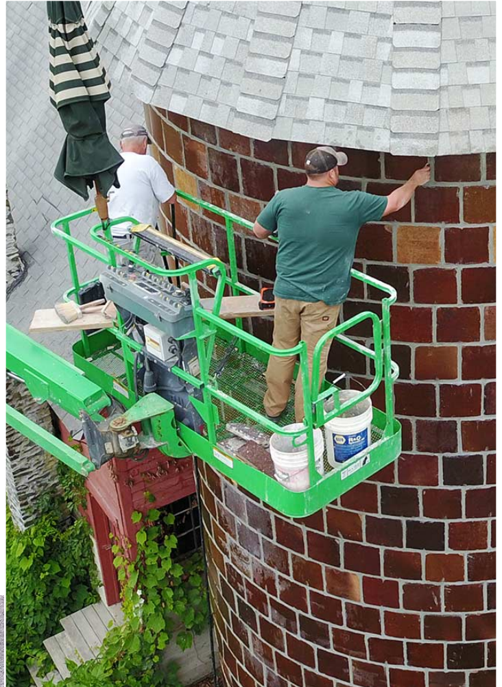
Below: Quonquont dairy barn silos tile and grout restoration, 2022
