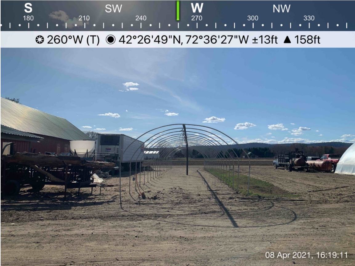
Image 2: Looking west at location of damaged/removed greenhouses in existence on April 24, 2018 within A/R-1.
