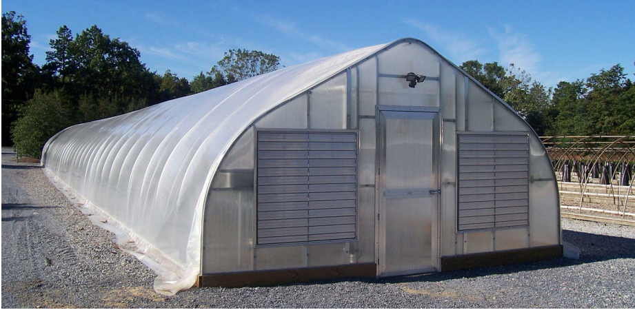
Source: Rimol Greenhouse Systems
