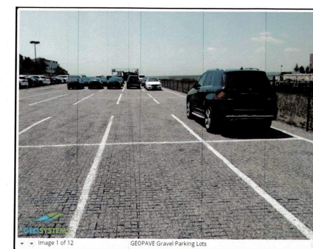
12 POROUS AGGREGATE PAVING EXAMPLE NOT TO SCALE
