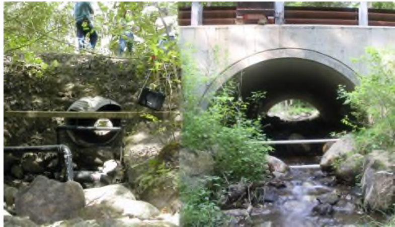
Culvert replacement on Mitchell Brook (Scott Jackson)
